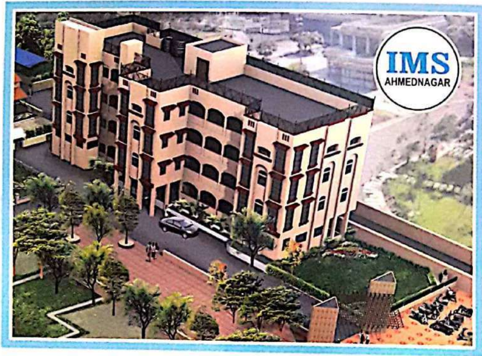
IMS - MAIN BUILDING
